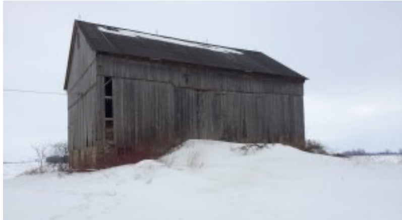
Rural ON Barn - Picture provide by the Ontario Barn Preservation
